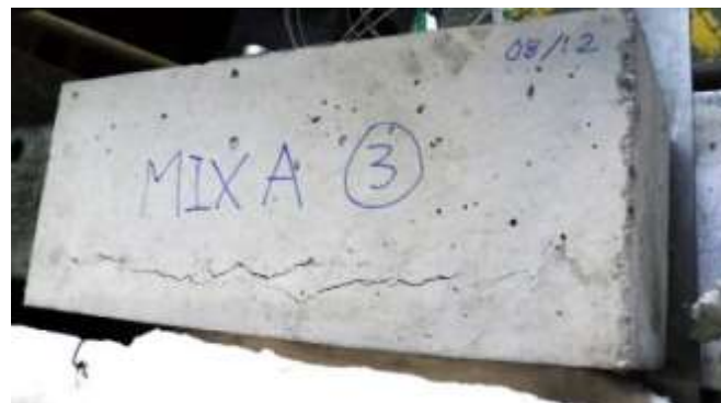
Figure 4. Large crack on top of specimen PC3
